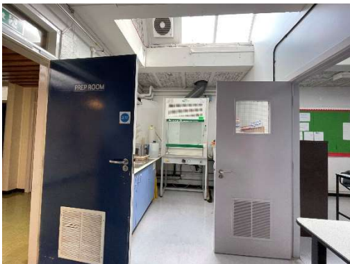
Figure 19 A door from the main prep room into one of the classrooms with no door closer installed
