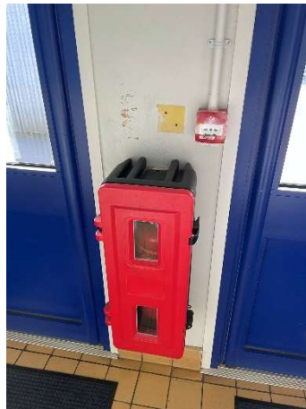
Figure 10 An example of missing signage by fire equipment
