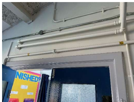
Figure 10 An example of missing signage by fire equipment
