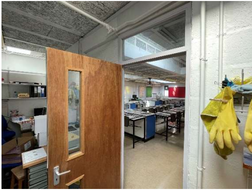
Figure 19 A door from the main prep room into one of the classrooms with no door closer installed
