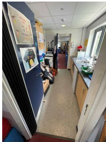
Figure 24 The fire doors in the music room propped open during the night
